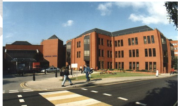
Entrance to Lincoln Wing at St. James's University Hospital
